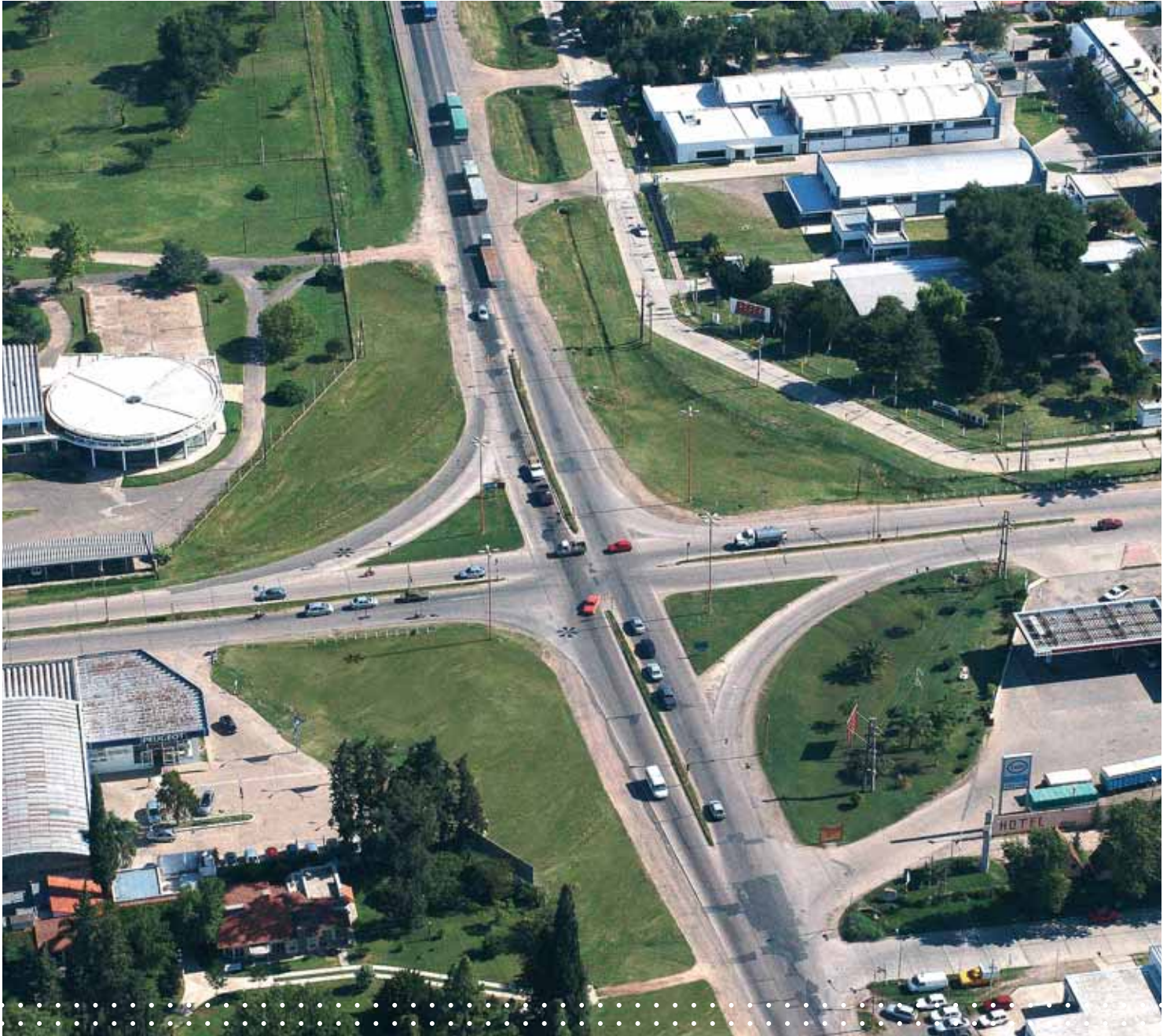
VISTA AÉREA. CRUCE RUTA NACIONAL 34 Y RUTA PROVINCIAL 70. / AERIAL VIEW OF NATIONAL ROUTE 34 AND PROVINCIAL ROUTE 70 CROSSROADS.
